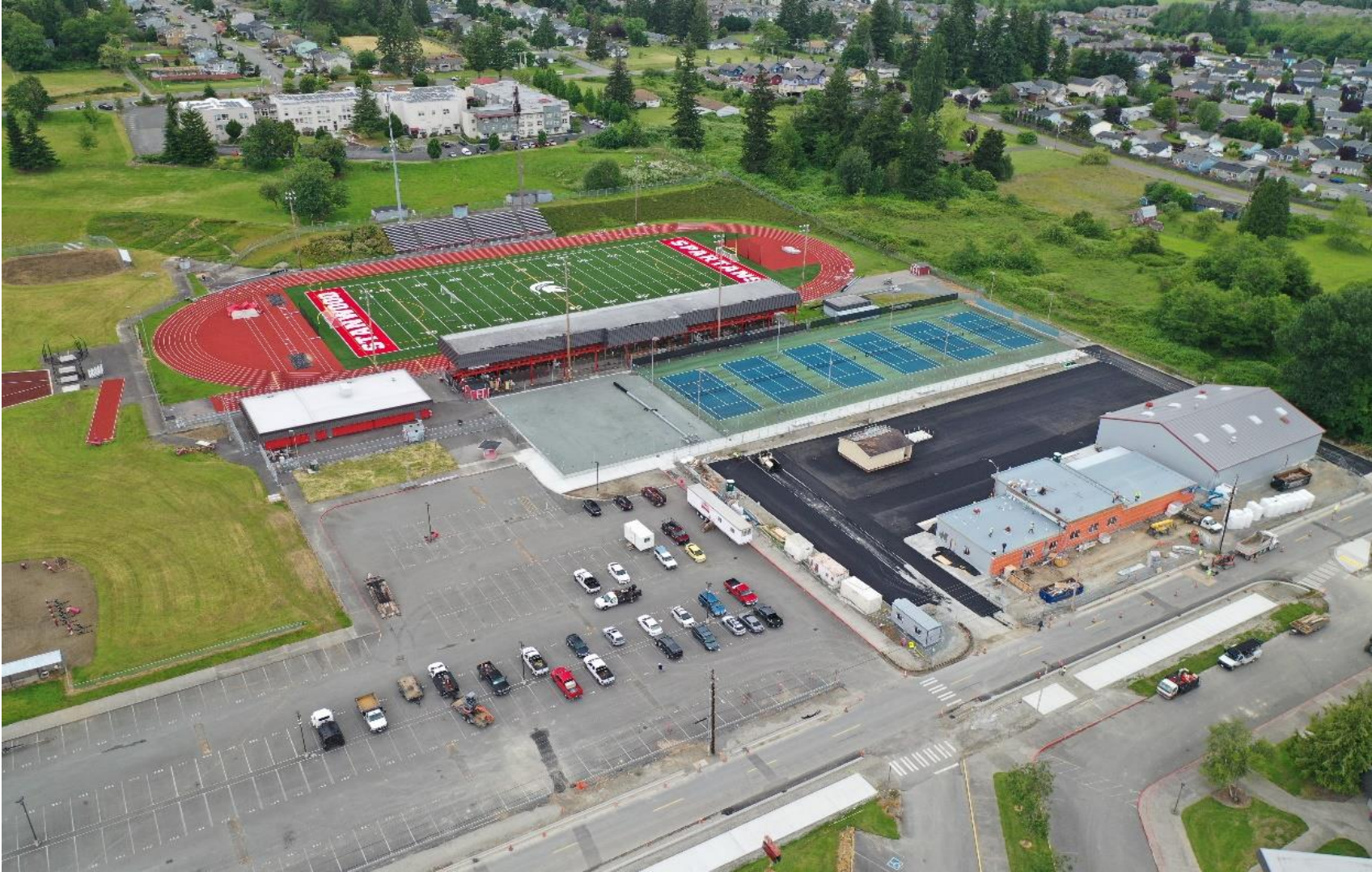
OVERHEAD VIEW OF MTC, TENNIS COURTS, STADIUM, FOOTBALL FIELD
